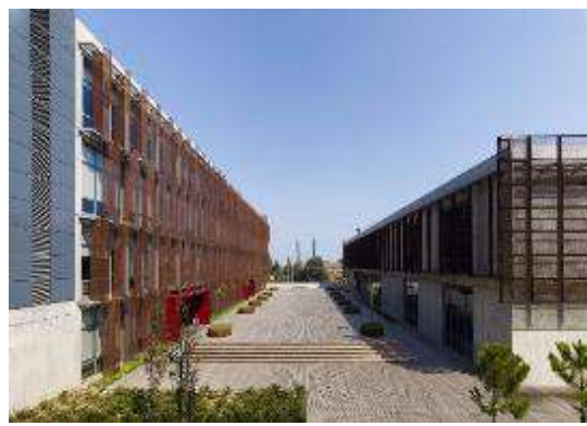
Figure 5: Usage of perforated corten plates
