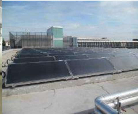
Figure 3: 120 solar collectors the roof
