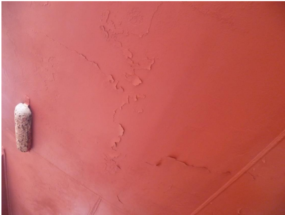
Figure 4.22. VESSEL 3, 2013 Dry-dock, photo of hull condition, condition after 1 st type self- polishing coating application with only %25 blasting
