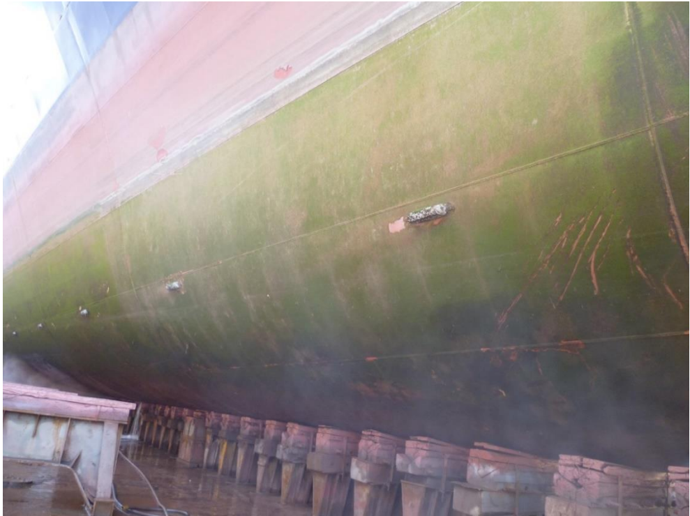
Figure 4.30. VESSEL 4, 2013 Dry-dock, photo of hull condition, condition just after entering the dry-dock
