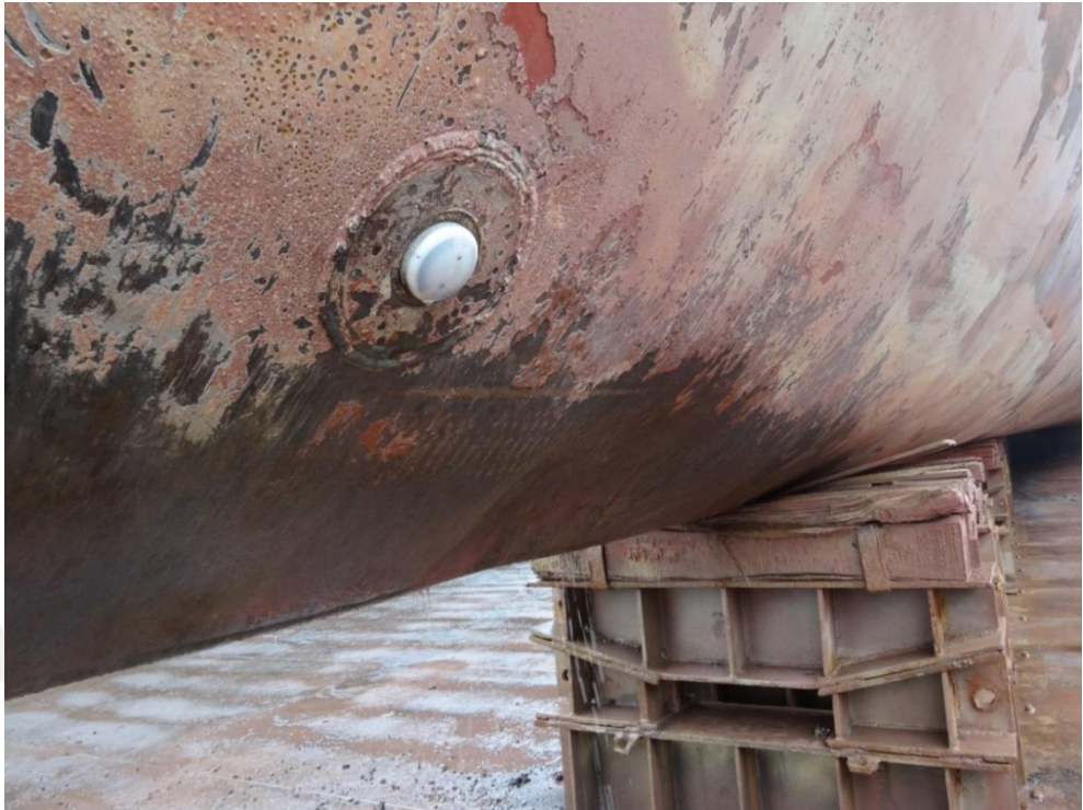
Figure 4.52. VESSEL 6, 2015 Dry-dock, photo of hull condition, after high pressure water wash
