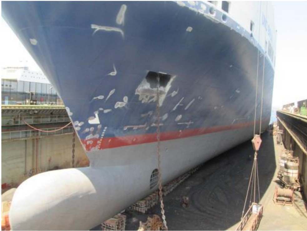
Figure 4.12. VESSEL 2, 2014 Dry-dock, photo of hull condition, after full blasting, condition before 1 st type foul release coating application
