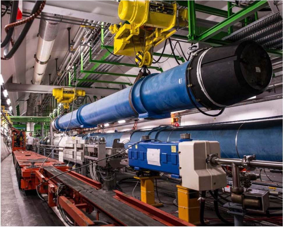
Fig. 5.13. Transfer of an LHC cryo-magnet between the transfer tunnel TI 2 (foreground/left, with the beam line arriving from the right) and the LHC main tunnel (background/right).
