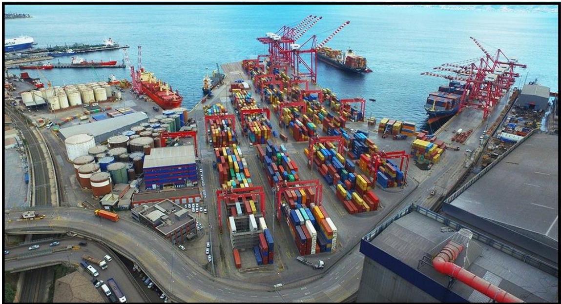
Figure 5.10. An Image from the Land Side of YILPORT. (Source: https://www.yilport.com/en/media/gallery/Gebze-Turkey/200/220/0 )
